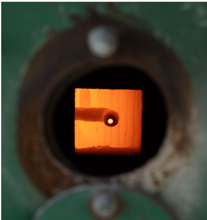
Picture: Combusted pyrolysis gas, providing heat for the asphalt drum dryer.
