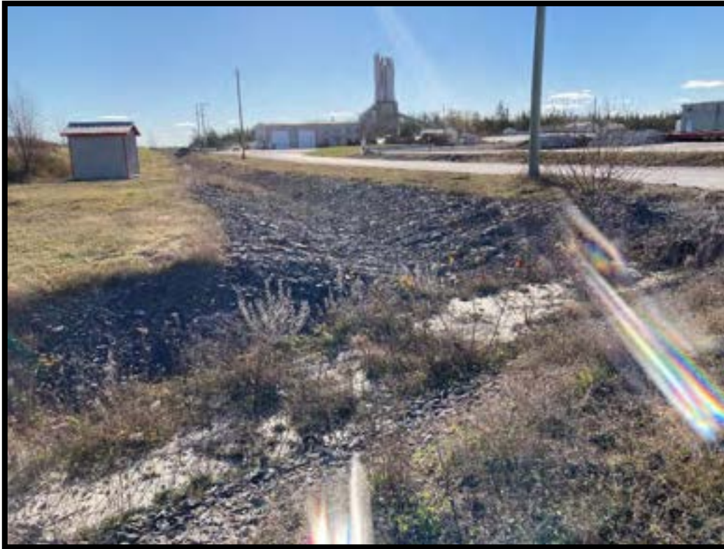
Figure 13: Drain, driveways, and buildings of active quarry. (MH1141-D001)
