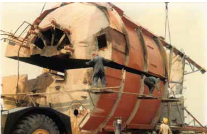
PHOTOGRAPHED ABOVE: Large tower being cut in half to be transferred from Bourget to the new Cumberland Ready Mix plant.
